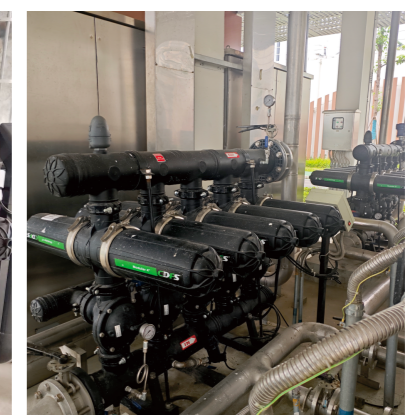
Reclaimed Water Plant Project
